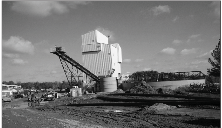
View of River Queen on-site coal processing facility during reclamation. Photo by AML
