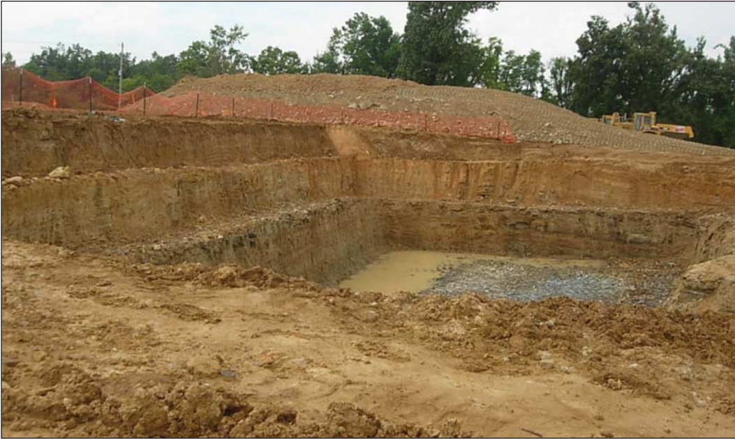
Excavation at the site to prepare for construction of the Ohio County plant expected to be completed in spring 2011.
