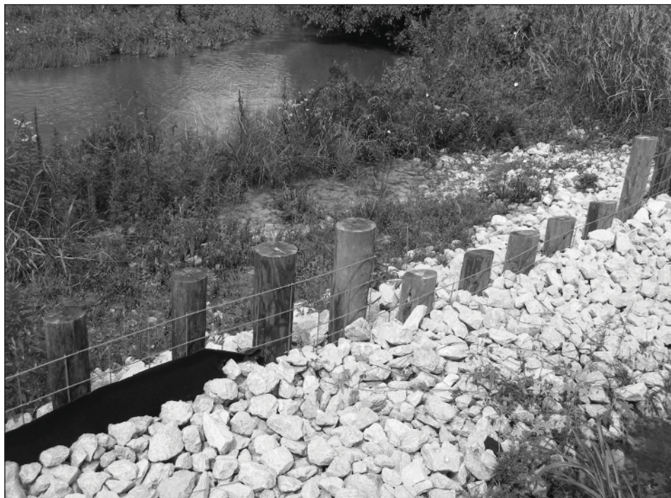
A large gully formed by high traffic near the stream was repaired and the area is now deemed a “no-mow” zone. Photo provided by the UK College of Agriculture
